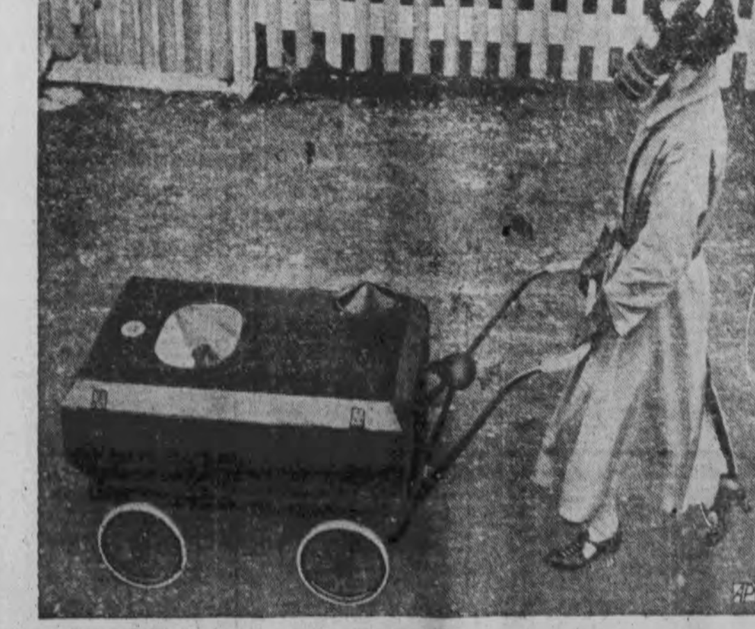
HUSH-A-BYE, BABY, GAS IS HERE, and that means mother will use carriage invented by E. W. Mills. A cow-protected filter fits in the lid. Squeeze of bulb pumps in fresh air.
