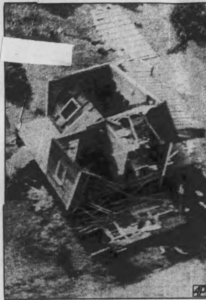
The wreckage shown here is all that remains of a Charleston, S. C., residence that was in the path of the furious tornado that struck the historic "City by the Sea," killing 28, injuring 200 and doing unestimated property damage.
