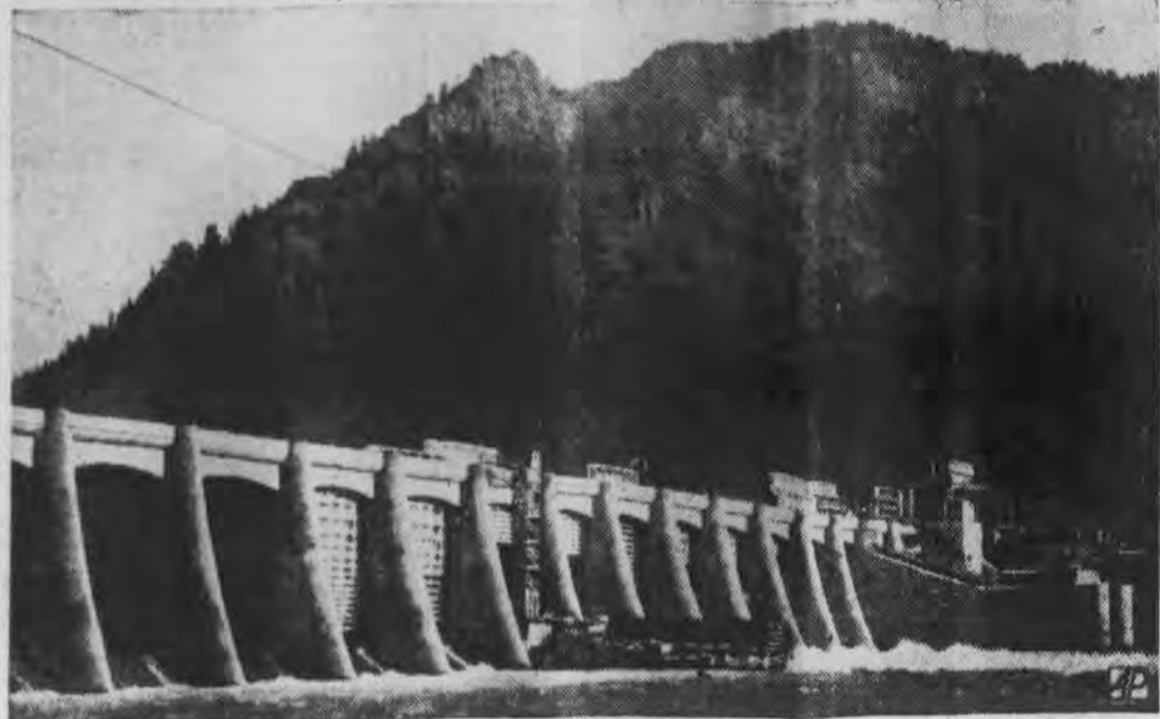
IT PROVIDES FOR FISH The Bonneville dam, a section of which is shown, cost $52,000,000, provides cheap power, makes in- land The Dalles, Ore., a seaport. Jutting downstream is a temporary fish ladder; on the far side, a permanent one. Salmon brood upstream for the spawning season, climb these.
