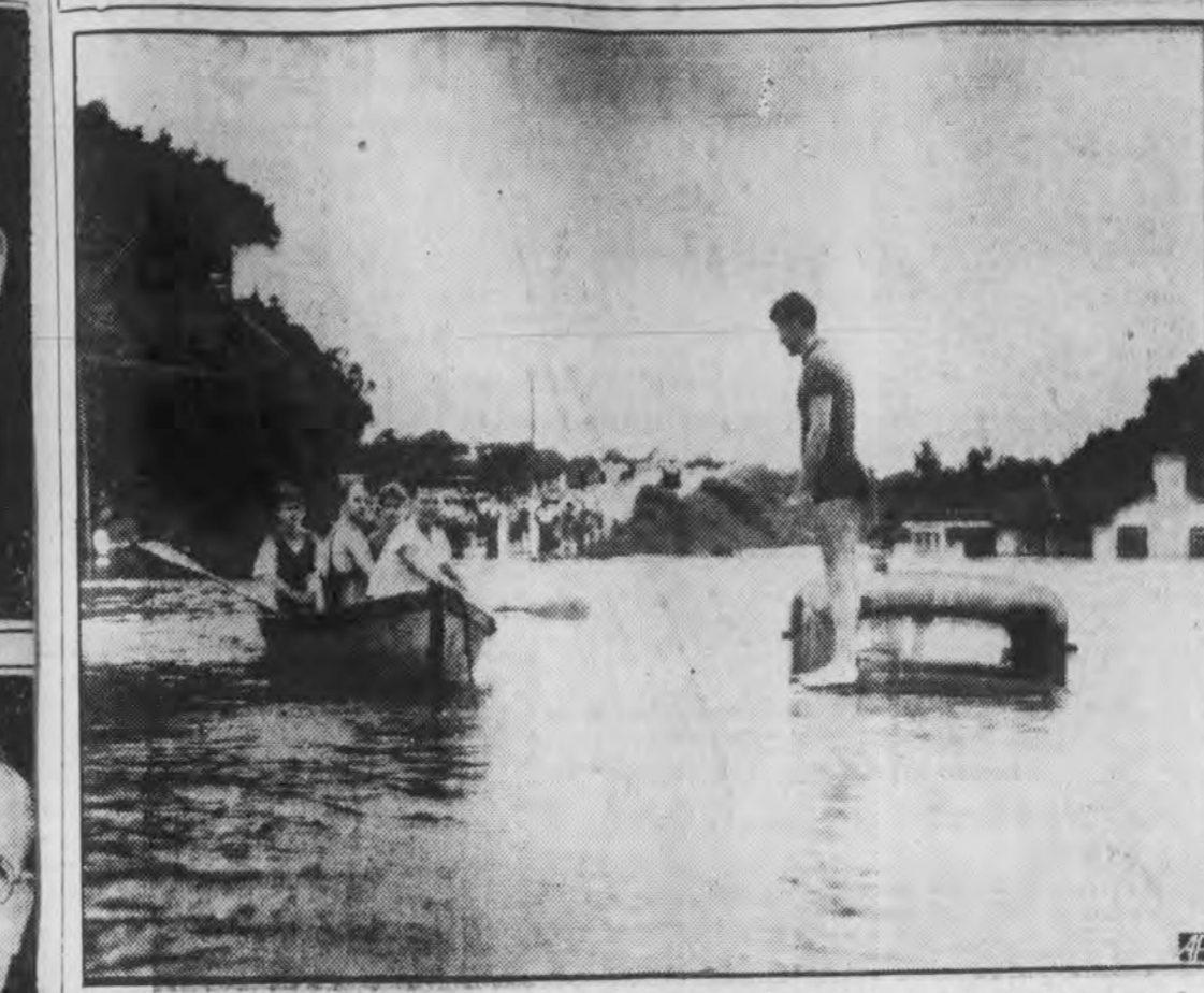
Six days of continual rainfall brought about conditions like this at Bethayres, Pa. Here a marooned motorist prepares to accept aid from a party in a rowboat on Route 232. Note people in the background who have been cut off from town by the submerged highway.
