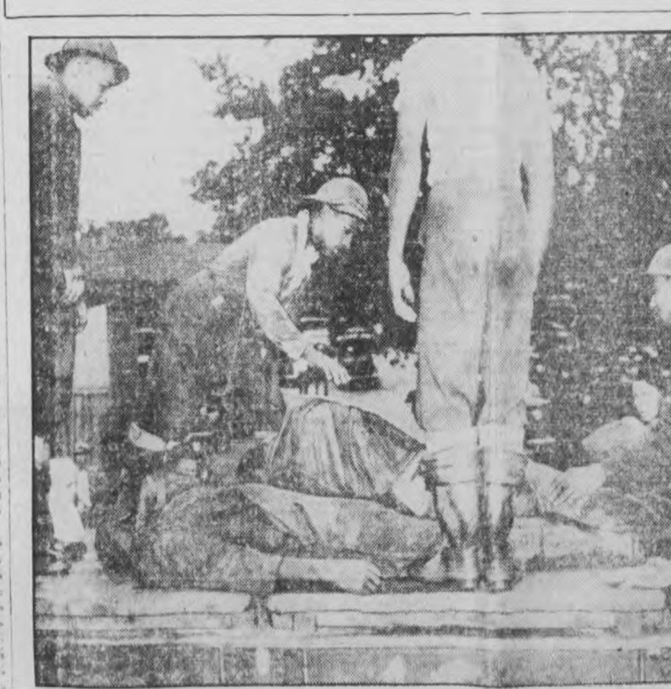
Eleven workmen were killed and four others were injured by a dynamite blast in a water tunnel under construction far under ground at Baltimore. Rescue crews are shown bringing the bodies to the surface and laying them out to a wait identification.
