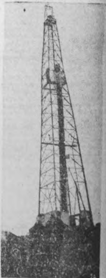
TO FIND OIL , Anglo-American company engineers drilling near Dalkeith, Scotland, went down more than 1,800 feet. Interested Scots come to watch the boring operations.
