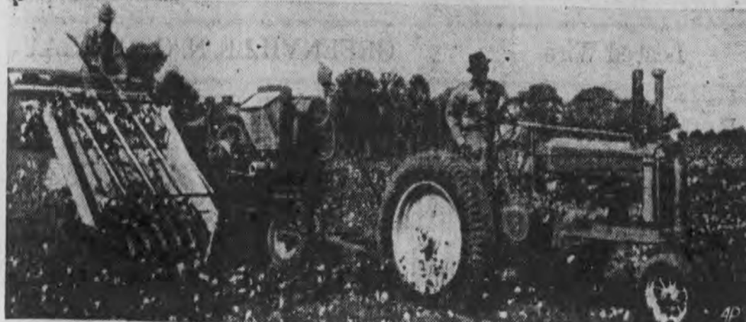
STALK & CO. This cotton harvester, made to garner the whole plant, cuts and dumps the harvest in 150-pound bales ready for the market. By-products from stalks means extra profit.
