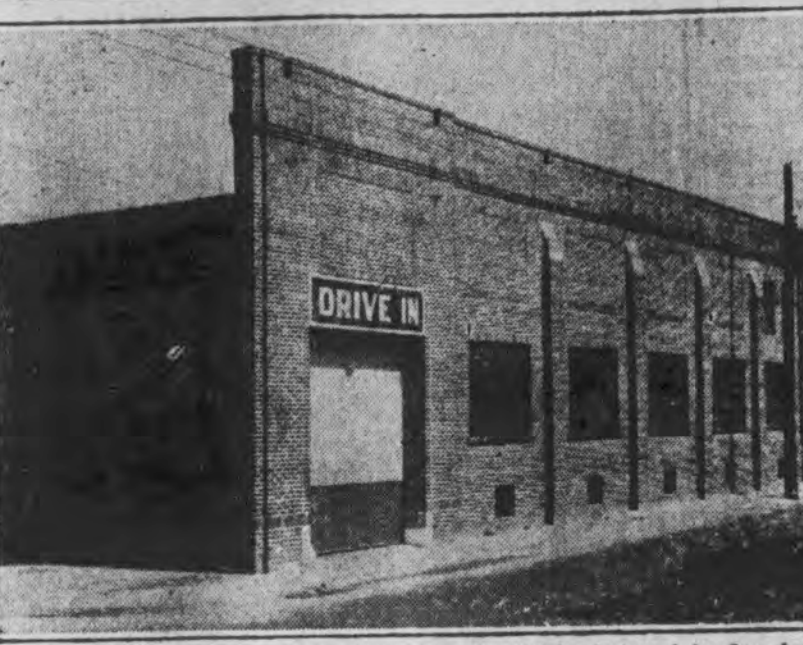
Webb's tobacco warehouse, shown above, was completely destroyed by fire shortly after noon today from undetermined origin. Even before the blaze was burned out, owners announced that the structure would be replaced. Smith and Sugg had leased the warehouse for this season and are expected to occupy the new building.
