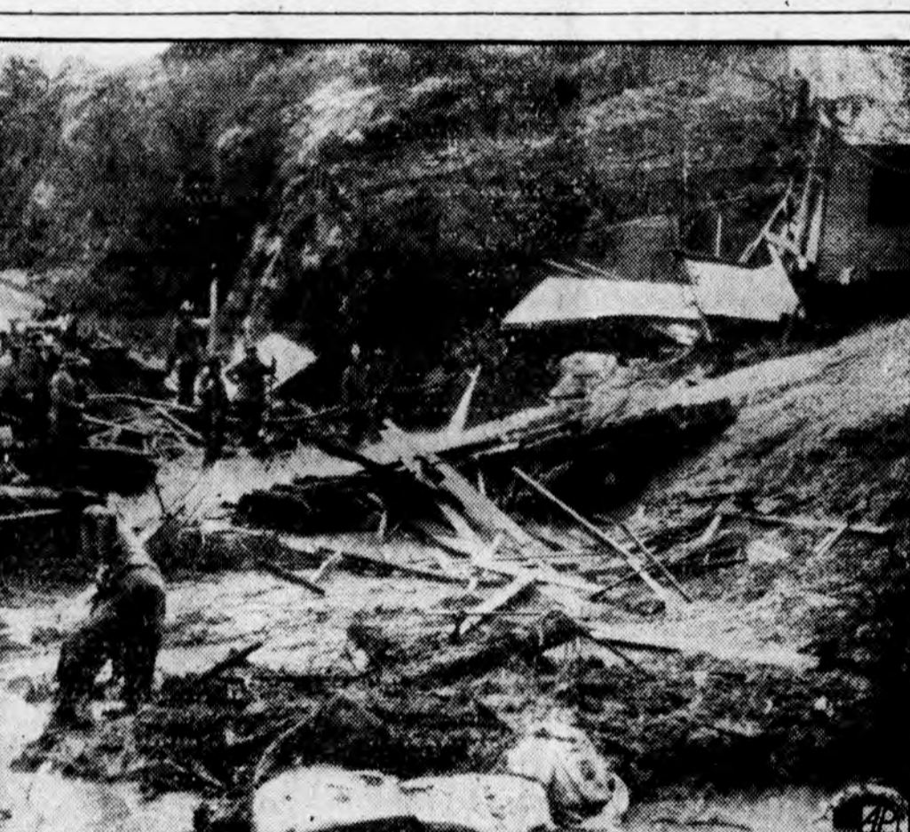
Leonard Randall, 6, perished and his mother, Mrs. Joseph Randall, was reported buried in debris when their hillside home, caught in the grip of a thundering landslide at Los Angeles, crashed into another residence (upper right) and collapsed. The landslide was precipitated by heavy rainfall; and scores of persons were reported dead or missing as floodwaters marooned parts of Los Angeles and nearby communities. Here firemen hose away mud and debris hunting for possible victims of the Randall home collapse.
