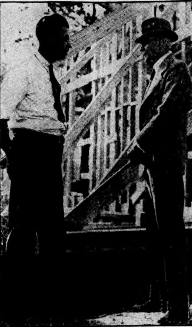
Even when he is taking a winter vacation on his plantation at Ways, Ga., Henry Ford, the automobile manufacturer, remains busy. He is seen talking to one of his employees (left) in front of a new building being erected.
