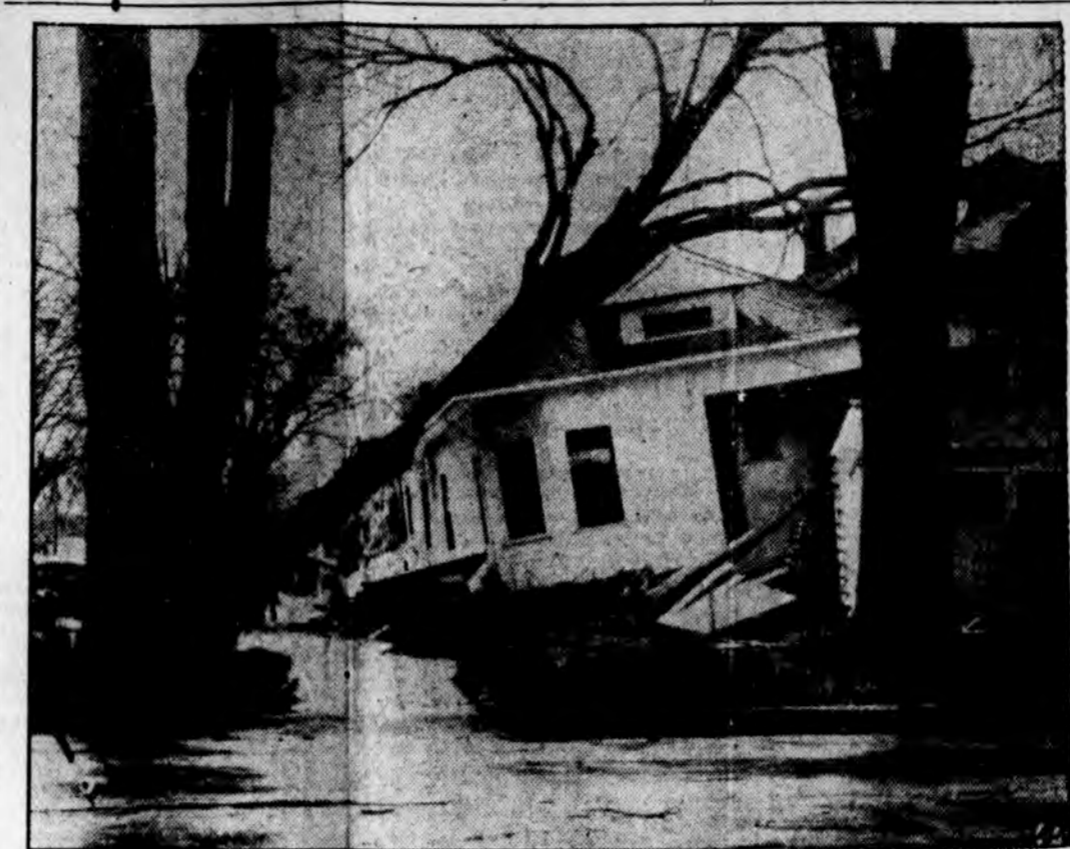
Five persons were killed and scores of others injured when a hurricane, reaching in spots almost tornado force, swept through northern California causing property damage estimated at millions of dollars. This Sacramento scene shows how a 45-mile an hour wind, using an uprooted tree as a lever, ripped a house off its foundation and jammed it into its neighbor.
