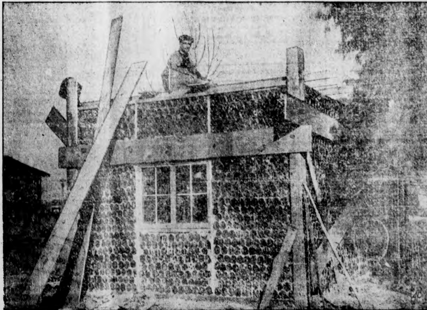
WHAT TO DO WITH OLD OIL CANS was readily answered by canny Albert Baker of Phoenix, Ariz. He collected some 8,000 oil cans discarded after their contents had been used to lubricate motors and used them to build the walls of his new home. He plans to cover over the cans with plaster, when the framework is completed.
