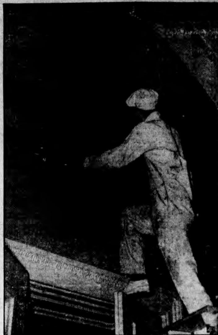
...COMPLETING THE SETTING for what may prove an historic meeting of American legislators, this painter adds the final touch to the great seal. Others replace carpets, repair furniture, scrub and paint, while still others will install an air conditioning system.
