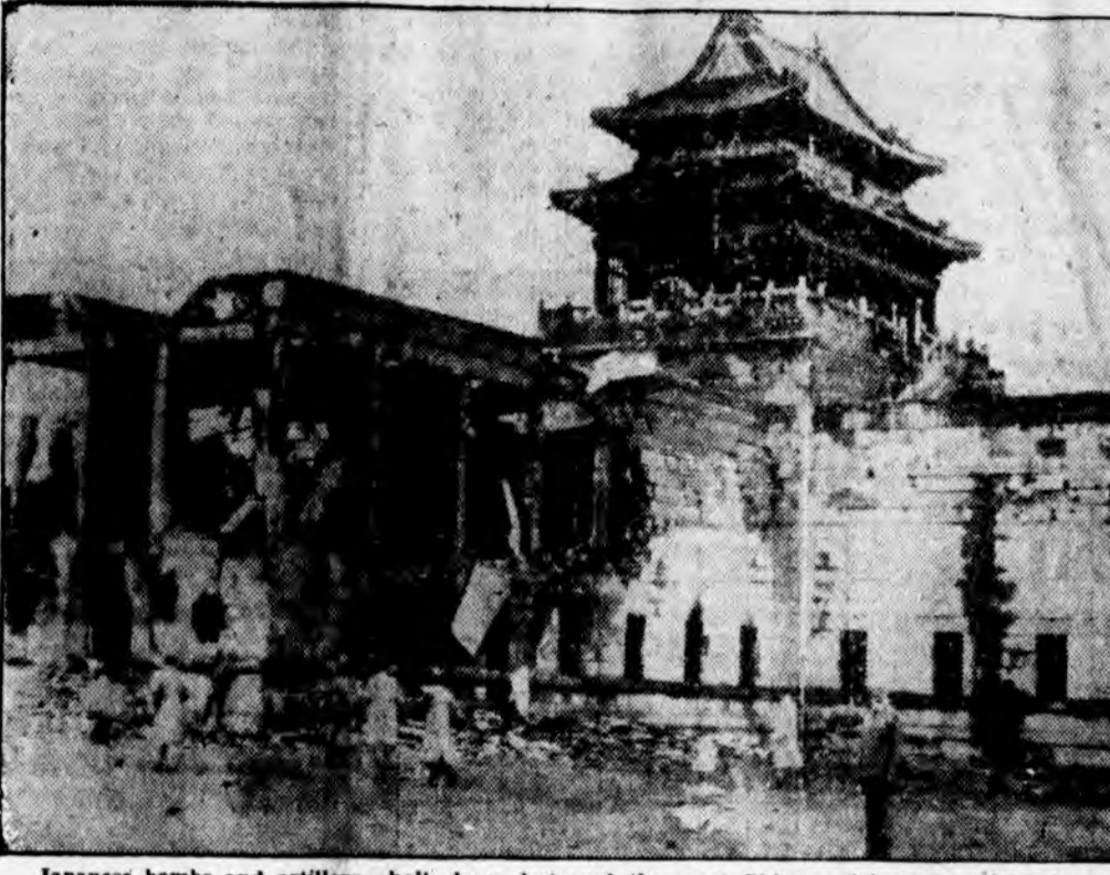
Japanese bombs and artillery shells have destroyed the great Chinese civic center which housed the municipal government of greater Shanghai. Administration buildings, hospitals, library, museum and the athletic stadium were among the structures shot to pieces. Among those who inspected the ruins shortly after the shells stopped falling was James A. Mills, Associated Press war correspondent, who is seen standing (right) in front of the bomb-wrecked building.
