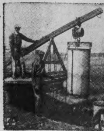
PUBLIC-ENEMY TRAP The cylindrical contraption, called a lysimeter, is being planted by Oklahoma agronomists to find what force of nature steals nitrogen from the soil.
