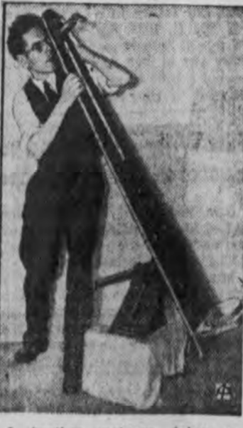
5—Another engineer takes a squint with the completed job. Stars are reflected from mirror at bottom to focus at top.
