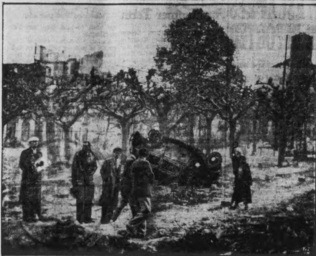
WAR'S DESOLATION. Centuries of tradition, of culture and time-seasoned beauty are crumbling ruins at Guernica, Spain, ancient capital of the Basques. Nearly every building bears evidence of bombs and bloodshed.
