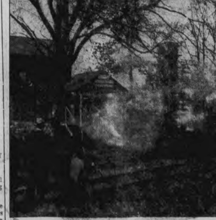
EXPLOSION—DELIBERATE. Dr. Price deliberately produced this blast in his Arlington, Va., "explosive gallery" to prove that dust explosions gather force as they go. This explosion was started under the shed in center but did not attain its full force until it reached the tower at right.
