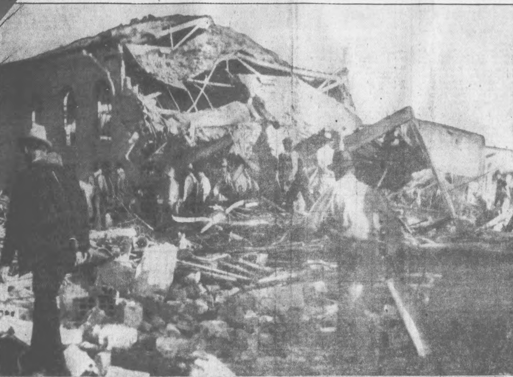
Rescue workers are shown searching the debris of the Consolidated School at New London, Texas, for bodies of hundreds of children and teachers who perished when a mysterious explosion wrecked the building. Four hundred and twenty-five bodies were recovered within a few hours after the disaster. School authorities at first feared that 670 perished. (Associated Press Photo—Copyright by Oklahoma City Daily Oklahoman.)
