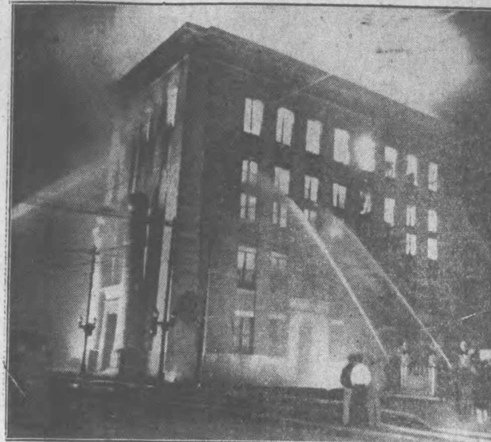
Bursting through the roof and windows almost in one spurt, $250,000 fire is shown destroying the Masonic Temple at Charlotte, N. C. Flying embers showered on three city blocks, but principal damage aside from the temple itself was confined to awnings. (Associated Press Photo).
