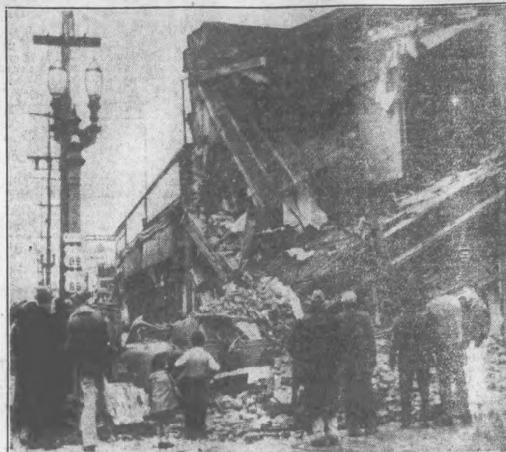
An automobile leaped the curb in Los Angeles, tore down a two-story building and tons of debris fell on the car in which three persons were riding—but nobody was injured. The car happened to strike a vital corner post supporting the building and it crashed in a flash. (Associated Press Photo).
