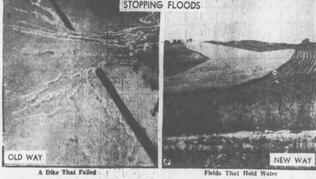
A Dike That Failed. Fields That Hold Water
