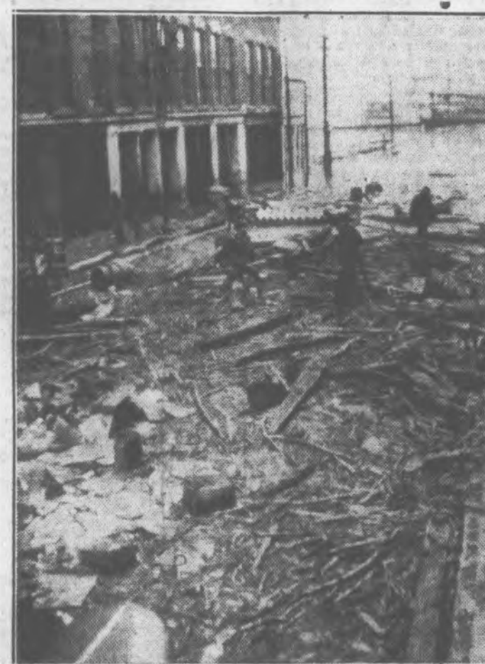
Here's a typical street scene in Louisville, Ky., as flood water receded from the city. No sooner had the muddy tide gone down than workmen plunged into the job of clearing the streets of the debris. (Associated Press Photo)
