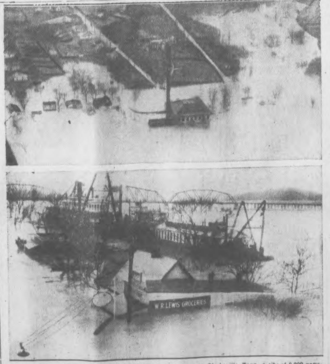
Surrounded on all sides by high water from the Cumberland river, Clarksville, Tenn., a city of 9,200 population, was left in darkness and the supply of drinking water was cut off by the inundation of the water-works plant and the failure of power lines. The water pumping station is shown (top) under several feet of water. Below houses in Clarksville are shown with water almost to the rooftops. (Associated Press Photos)
