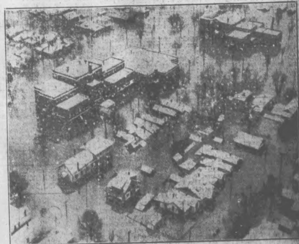
Among the cities hardest hit by the Ohio river flood was Jeffersonville, Ind., all of which was inundated. About half of the town's 12,000 population moved out. A section of the city is shown with water lapping at the eaves of buildings and surrounding a new $1,000,000 school house. (Associated Press Photo)
