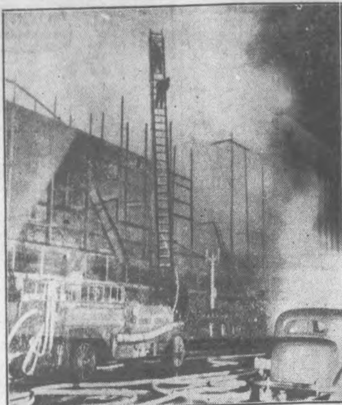
Perched on an extension ladder, firemen are seen playing a hose on flames which swept through a downtown business block in San Diego, Calif., causing $2,000,000 damages. A fireman and a seaman were critically injured before the spectacular fire was brought under control. (Associated Press Photo)
