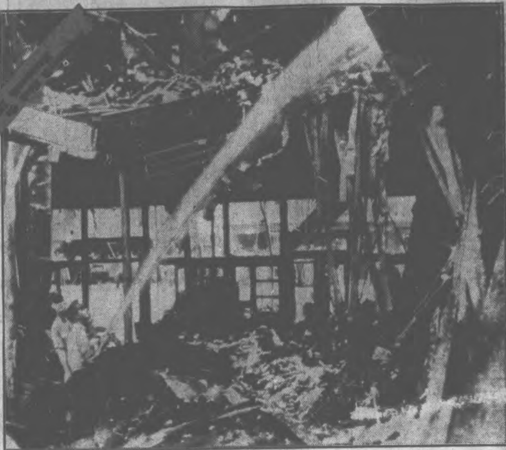
Five persons were injured, the nine-story Liberty bank building was partially wrecked and a fire spread to adjoining buildings was started by a mysterious explosion which jarred the downtown district of Waco, Tex. Damage was estimated at $275,000. Firemen are shown combating flames in the ruins. (Associated Press Photo)
