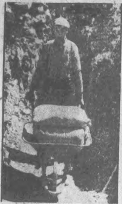
GOLD ORE MOVES OUT . . . A miner wheels out a load of gold ore from Jumbo, the hole in the ground where George Austin, 63-year-old hotel and store keeper in Jumbo, Nev., 40 miles away, struck it rich after paying only $500 down, with the promise of $9,500 later, for a claim.
