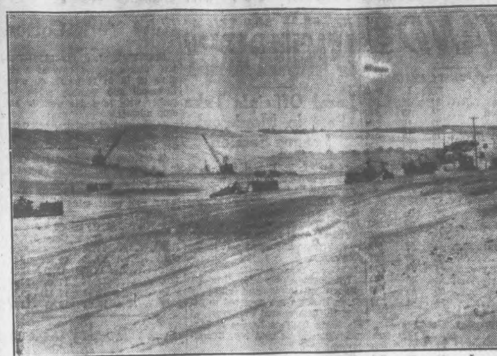
Here's a general view of the Florida ship canal near Ocala as work was being brought to a halt by lack of appropriations. Although actual digging is about to stop, engineering and geological surveys will continue. Camp Roosevelt, headquarters for workers, probably will be taken over—at least temporarily—by the University of Florida for extension work. (Associated Press Photo)
