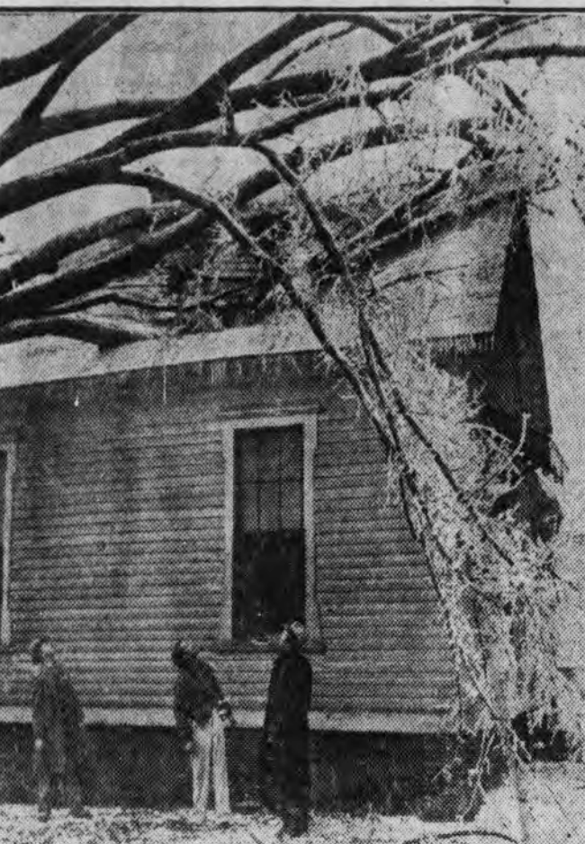
Here's one of the numerous houses damaged in Atlanta, Ga., when ice-coated trees broke and crashed down upon them during the worst winter storm the city had seen in a generation. Damage was estimated at $2,000,000. (Associated Press Photo)
