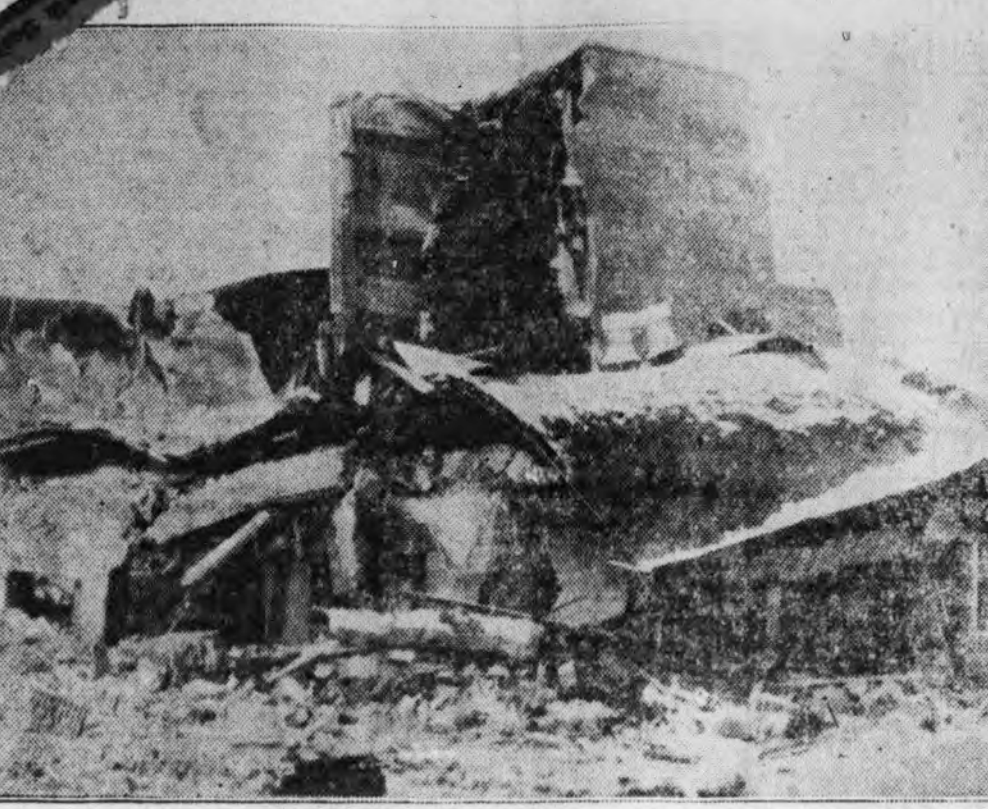
Two persons were killed and great property damage was done when the second earthquake in two weeks shook Helena, capital of Montana, during the series of tremors felt in 17 states and portions of Canada. This picture the wreckage of the Helena high school which was demolished completely. (Associated Press Photo).
