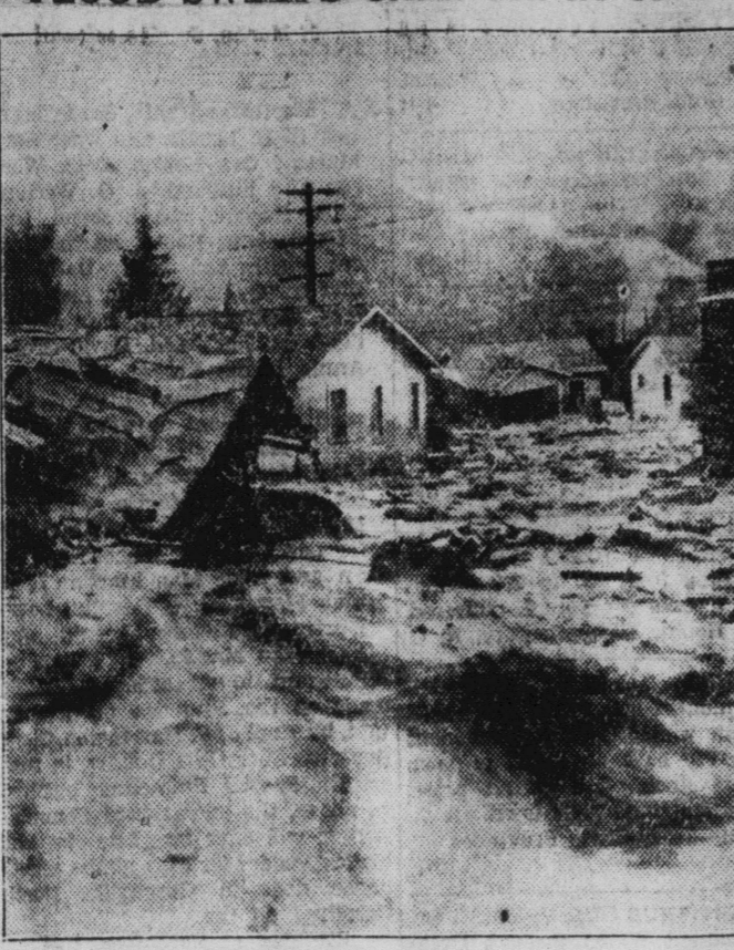
This is the second time this year that residents of Montrose, Calif., have had their homes wrecked by flood waters rushing down from mountain canyons. This picture shows what the flood did to the town. Montrose was struck by a flood of similar size New Year's day. (Associated Press Photo)
