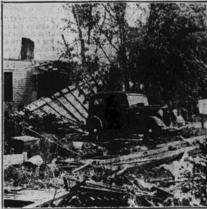
This automobile was left unscratched after the Jacksonville, Ill., tornado lifted its garage and sent it spinning into adjoining counties. Property damage in the Jacksonville storm was estimated at one million dollars. Several persons were injured but there were no fatalities. (Associated Press Photo)
