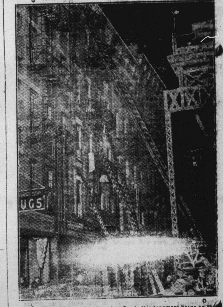
Seven persons lost their lives in a fire in this tenement house on the upper east side of New York, bringing to 25 the number of deaths from similar fires in the city in the last six weeks. The fire swept through the three upper floors of the building, trapping the seven. (Associated Press Photo)
