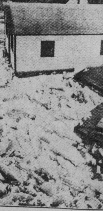
With the coming of warm weather, ice jams and floods are causing heavy damage in northeastern river valleys. Here is a scene on the Hudson river at Albany as boathouses, workshops and boats were crushed by the jam. Spectators said the whole surface of the river gave a mighty heave and tossed ice in all directions. (Associated Press Photo)
