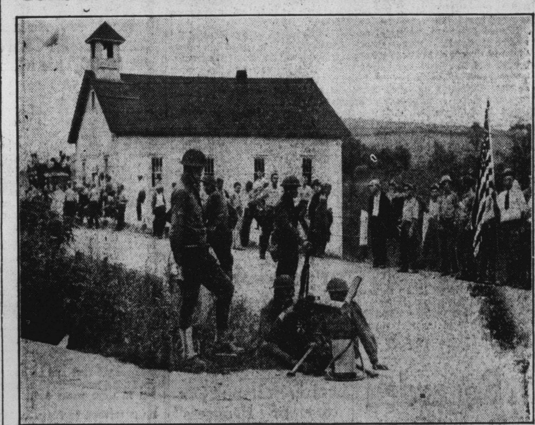
While both the state and federal governments moved for peace in Pennsylvania's soft coal fields, national guard machine guns frowned from hilltops and other vantage points in the trouble area. This picture was made on a road approaching a mine near Star Junction. While pickets watched sullenly from one side of the road soldiers were prepared for any emergency. (Associated Press Photo)
