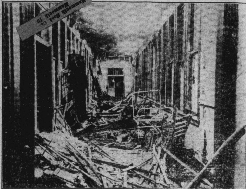
Rushed out on cots or carried down ladders, 226 patients were rescued when a fire swept the Robert Parker hospital at Sayre, Pa. A baby was born in the hospital when the fire was at its height. One of the damaged wards is shown above. The loss was estimated at $1,000,000.
