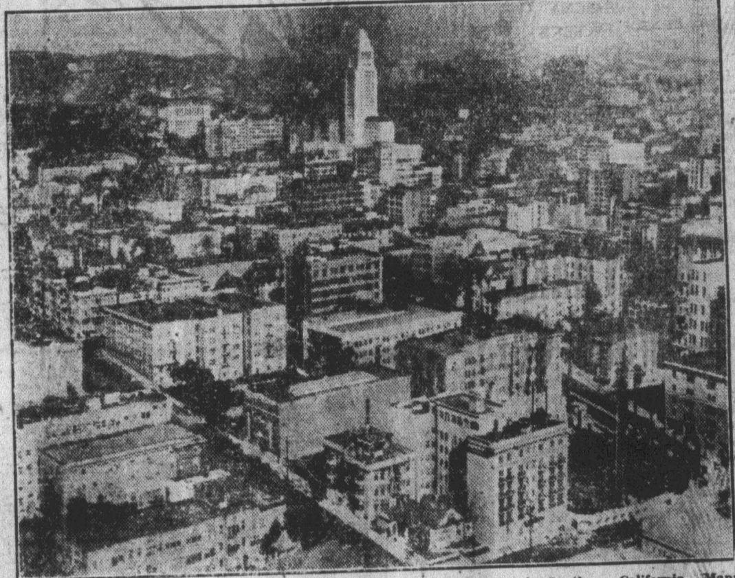
Los Angeles was one of the worst sufferers in the series of earthquakes in Southern California. Many of the city's buildings were damaged or destroyed and casualty lists mounted as new shocks jarred the area. This is a general view of the city looking over the business district before the earthquakes. (Associated Press Photo.)
