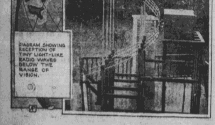
Guglielmo Marconi, delving into the mysteries of tiny waves only centimeters in length, has found that they follow the curvature of the earth to a certain extent, as indicated by sketch. The special herringbone like reflector antenna shown above was developed for simultaneous reception and transmission.
