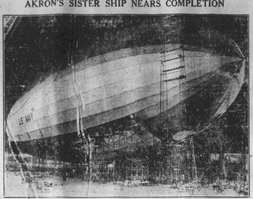
The huge U. S. S. Macon, sister ship of the giant Akron, is virtually completed. All fuel tanks have been installed, two of the four fins are in place, and instruments in the control car soon will be installed.
