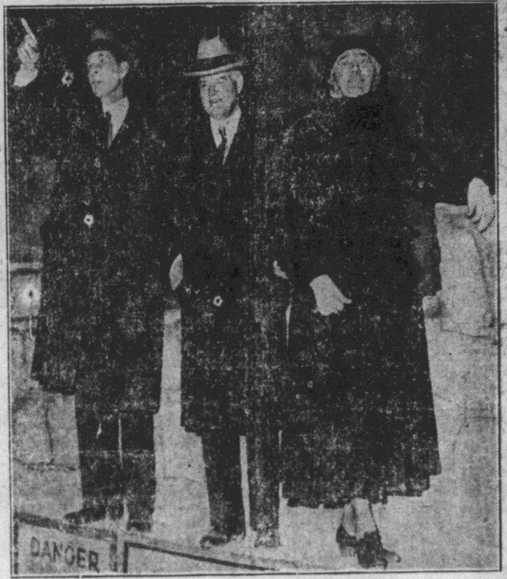
President Hoover inspected construction progress at Hoover dam, the gigantic project along the Colorado river, on his return trip to Washington from California. Secretary of the Interior Wilbur (left) is shown with the President and Mrs. Hoover. (Associated Press Photo)
