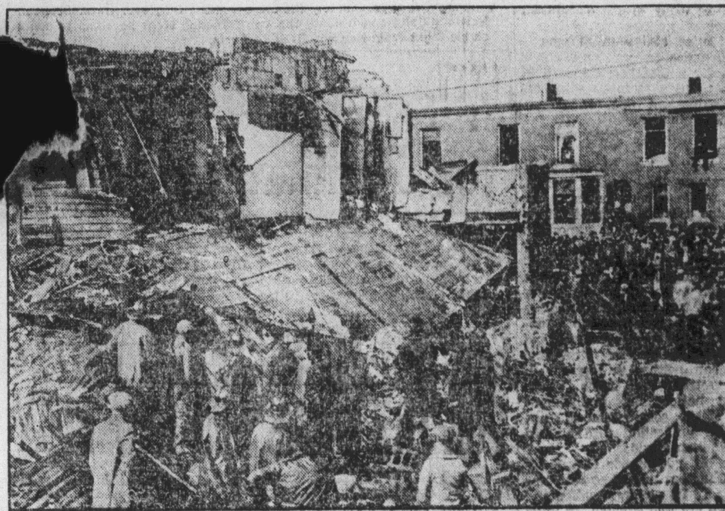
One person was killed and 24 others injured, several seriously, when a gas explosion in a Detroit plumbing shop wrecked four store buildings and a flat in suburban Highland Park. The shop where the explosion occurred is shown here. A broken gas main was blamed.
