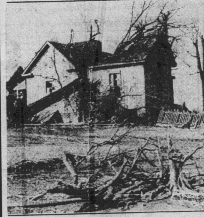
The above picture, taken in the heart of the storm area, shows a home cut in two by a tree blown against it by fierce winds of the storm which caused heavy property damage.
