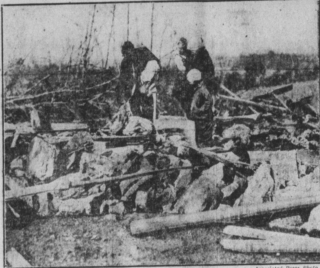
Associated Press Photo Lucky to be alive, the family of Gus Cannon returns to salvage a few belongings in the ruins of their home in northern Georgia after it had been shattered by a tornado's fury. Tornadoes left similar scenes of destruction in five southern states and killed more than 300 people.
