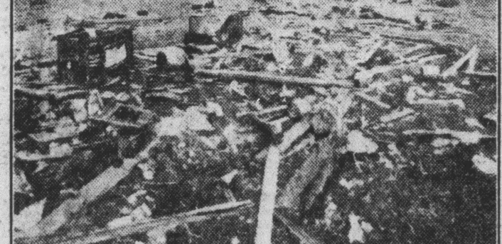
Two tornadoes in three days ripped across southern Arkansas killing three persons, injuring nearly a score and causing widespread property damage. Pictures show results of a tornado that struck Texarkana. A woman was killed in the wrecked house shown above. Below is the scattered remains of another house that was completely destroyed by the twister.
