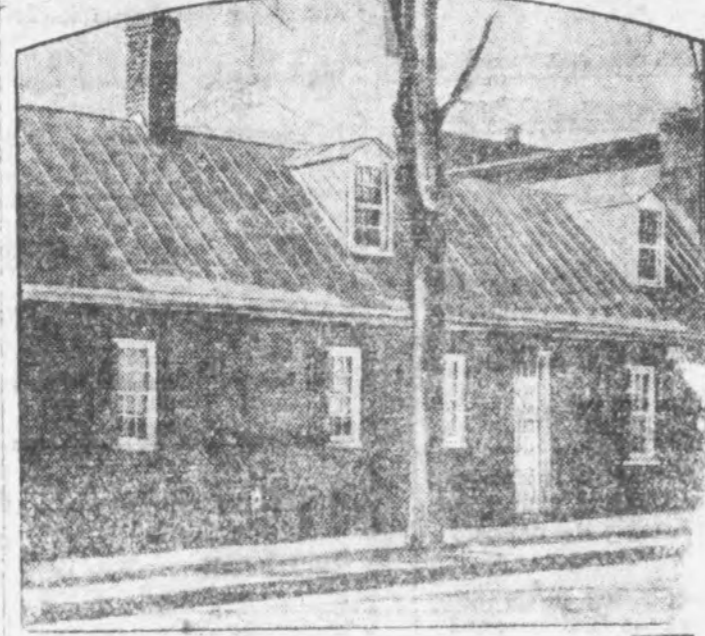
Virginia will receive from descendants of James Monroe (above) at Fredericksburg on April 25 the brick building in which the fifth President first practiced law. With it will come many relics, including the brass-inlaid desk (right) on which traditions say Monroe penned the Monroe Doctrine.
