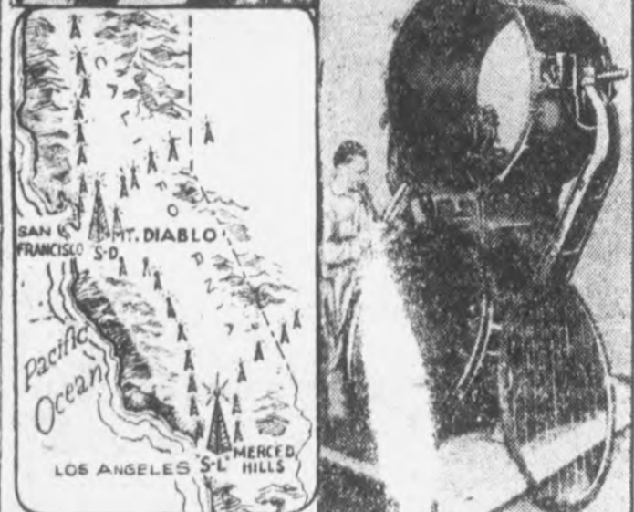
On Mount Diablo (above) and one of the Merced hills in California are being built two giant air beacons for night flyers which will be visible for 100 to 150 miles. The map shows their relation to smaller beacon lines projected or in course of construction. One of the huge lights is shown at the right.
