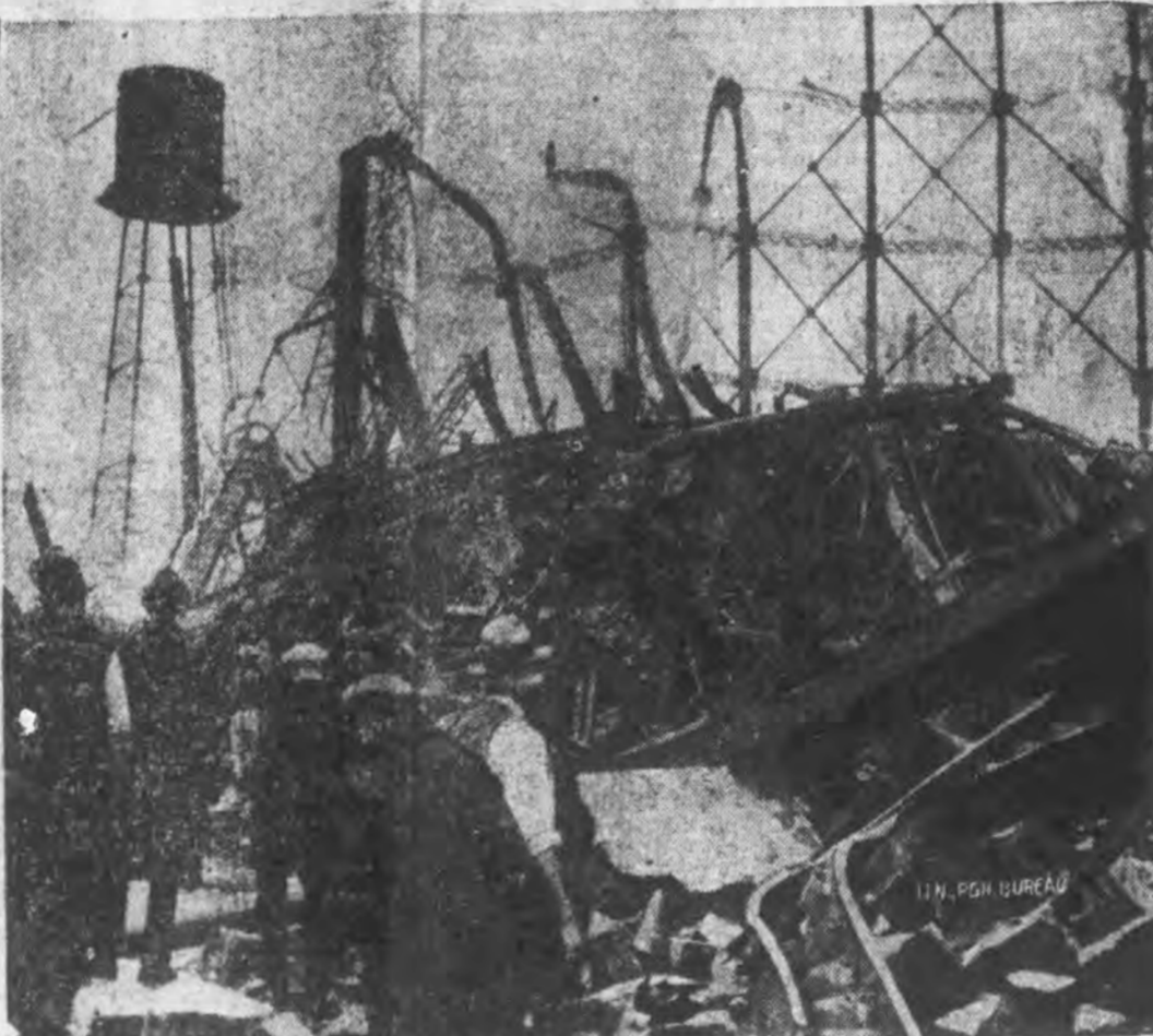
General view of wreckage of Equitable Gas Company plant in Pittsburgh, where many were killed and hundreds injured when huge storage tank exploded.
