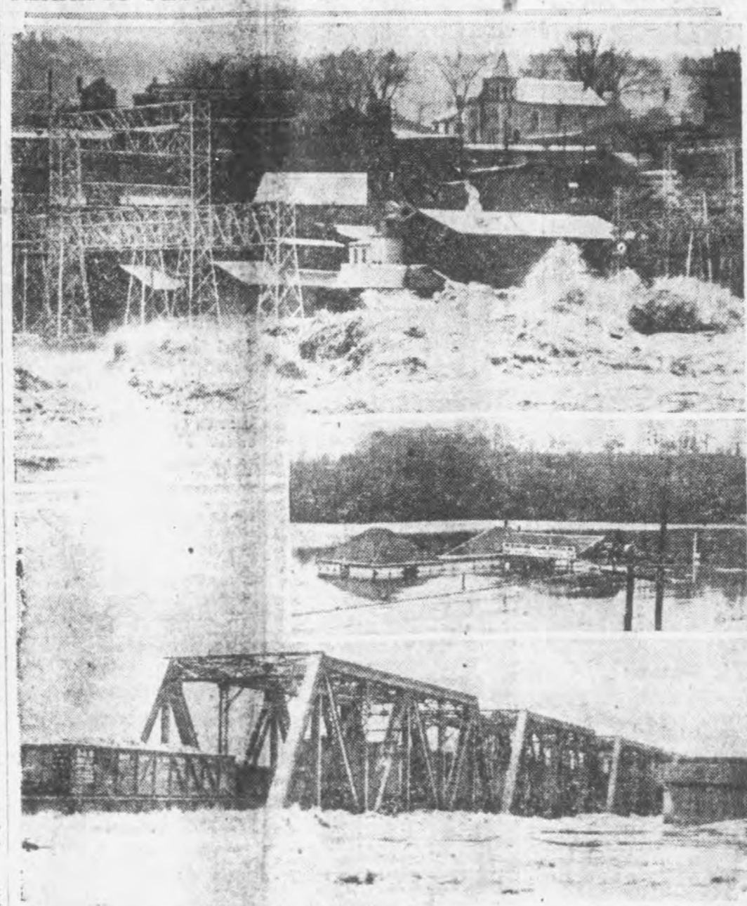
Billions of dollars in damages have been caused by torrents and bursting of dams in four states, hundreds of homes being swept away. Top: The raging Connecticut River flowing past Bellows Falls, Vt. Center inset: Inundated highway between Westfield and Springfield, Mass. Bottom: Floods raging over spot where dam was swept away at Bellows Falls.
