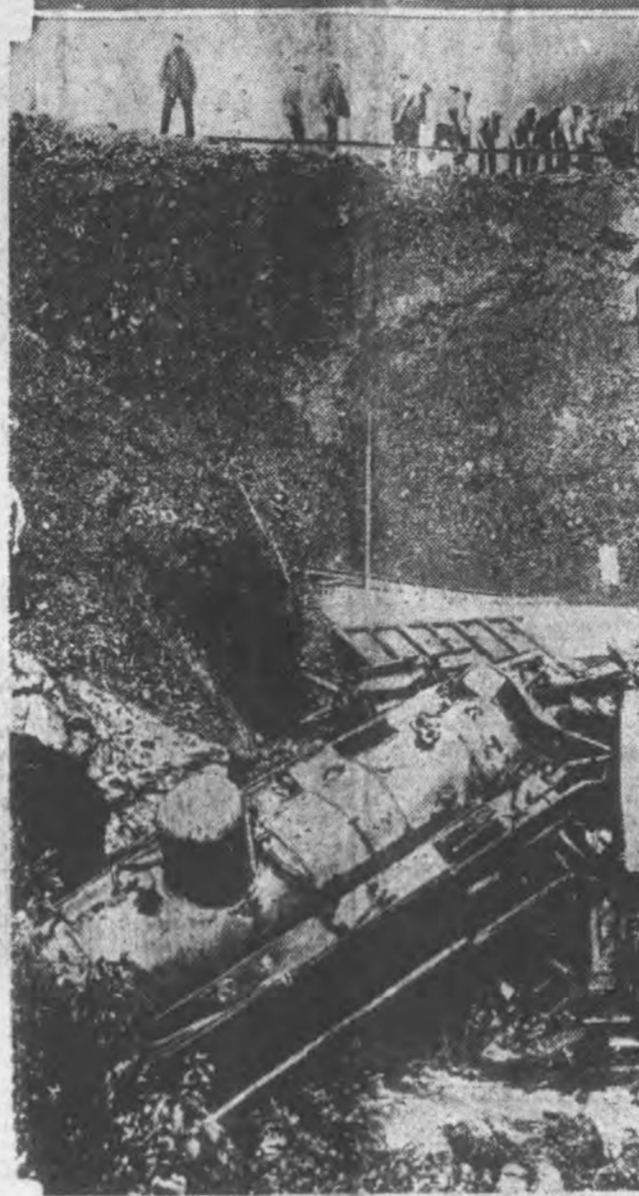
Here is one consequence of the disastrous floods now raging in Germany. High waters undermined railroad tracks at Wernigerode, causing a passenger train to plunge over an embankment. Nine were killed and twenty-two injured. Photo shows the wrecked train.
